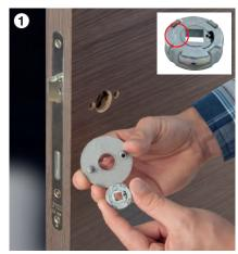
Please make sure to clip in the spring cassette in the right direction (the arrow indicates the handle's direction of operation).
