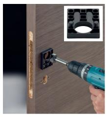
Drill the bore by using a standard Forstner bit (28 mm diameter) and the drilling jig available from HOPPE for the spring cassettes of flat handle roses.
