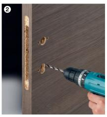
Drill the holes for the guiding lugs (remove the lock case for this).
