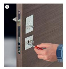
Fix the template on the door by inserting the key into the keyhole and mark the bores for the guiding lugs.
